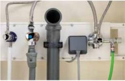
Cleanly and clearly mounted: cold and hot water, sink drain, surface-mounted socket, connection for drinking water pipe (e.g. for a coffee machine with a fixed water connection or a refrigerator with an ice cube make).
